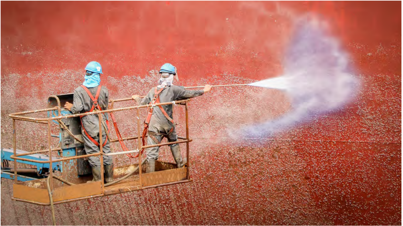
Figure 3.1 Removing biofouling by high Pressure Water Jetting. Source: Tawansak/Shutterstock.
