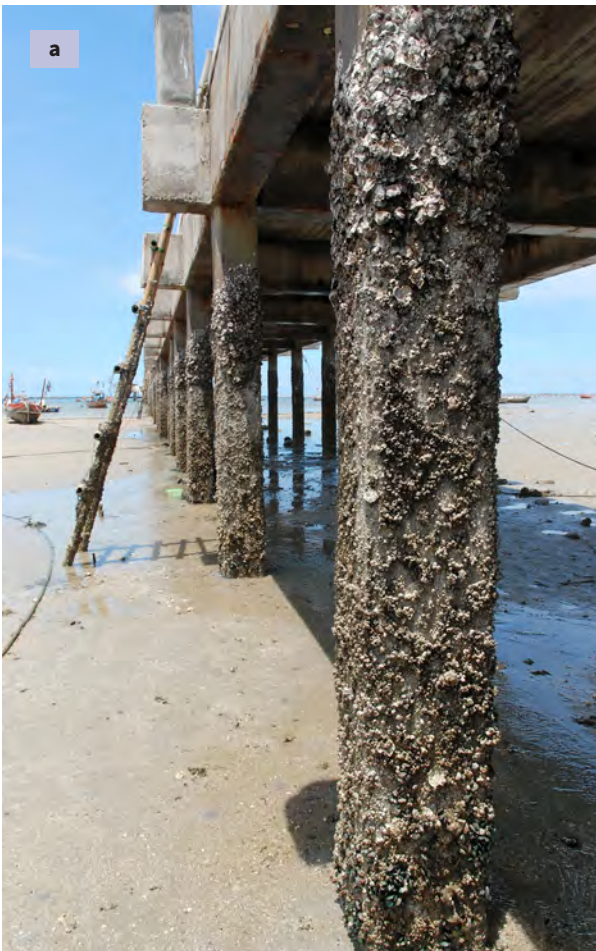
Figure 2.4 a) A concrete marine structure with severe biofouling. Source: Vorathep Muthuwan /Shutterstock.com; b) Mussels on a pier pillar. Source: Mikeledray/Shutterstock.com
