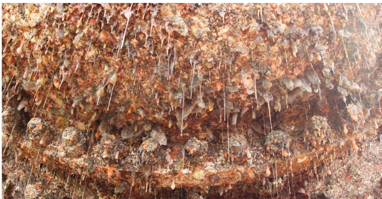
Figure 4.33 Biofouling on infrastructure deployed at the full-scale wave test site at the European Marine Energy Centre, Scotland (UK). Source: Andrew Want.
