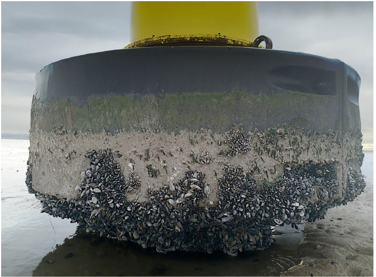
Figure 25. Cautionary buoy with biofouling (dominant species include Mytilus edulis , Semibalanus balanoides , Elminius modestus (IAS), Fucus serratus , and Ulva intestinalis ) in the Irish Sea.
